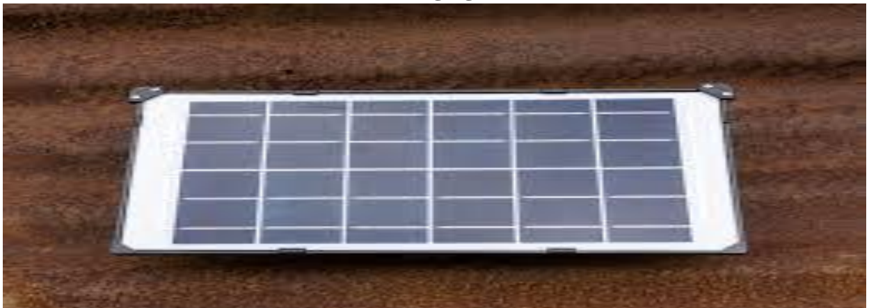
Solar Panel (Installation Phase)
