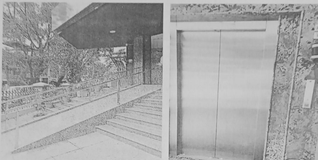
Figure 4: Common Facility – Ramp and Lift
